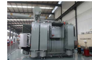
15MVA oil transformer adopt anti-corrosion design, C5-M painting, used for offshore
